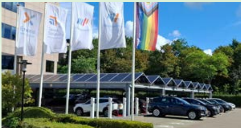
New solar panels at our Netherlands offices help power EV charging stations
